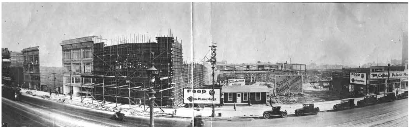
This wide-angle photograph shows the construction of the Crystal Palace Market in 1922. The street along the left bottom is Market; Eighth Street is along the right. Courtesy of the San Francisco History Center, San Francisco Public Library
