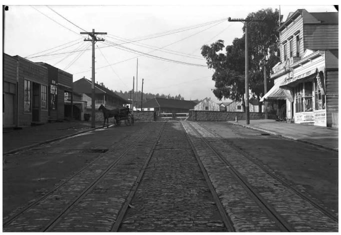
Cable trains ran into the Presidio over this track on Greenwich Street from 1892 until 1906. Note the gap in the Presidio wall and the off-center cable slots. Photo courtesy of SFMTA.
